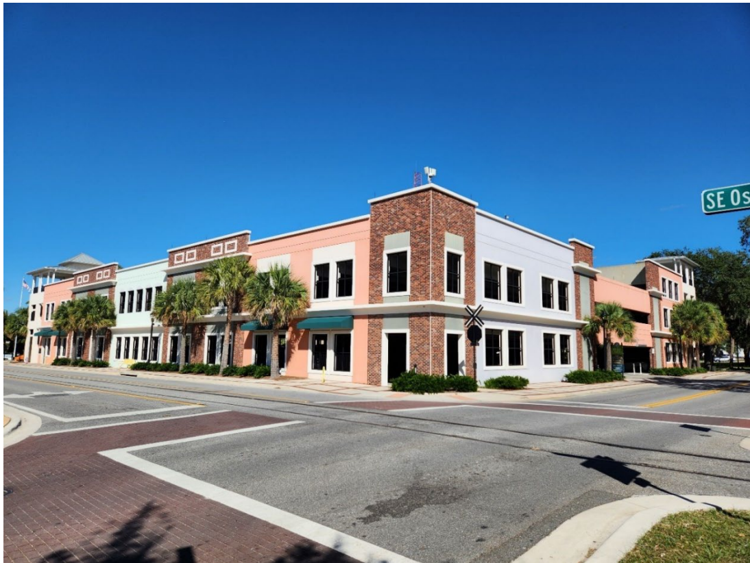
Figure 1. Parking Garage No. 1 - Intersection of E. Ft. King and SE Osceola Ave.
